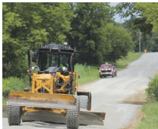
Photo Credit: The County Press, paving of a limestone road.
